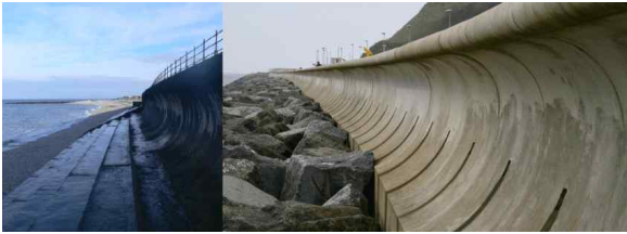
Fig. 1 Typical examples of a curved-faced seawall (from Castellino et al., 2018)
