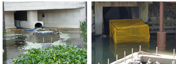
(a) Inlet (b) Outlet (exit of fishway)
