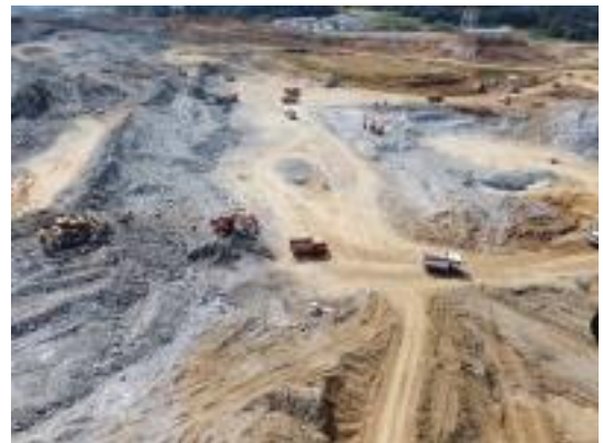
Fig. 3. Background condition of construction site
