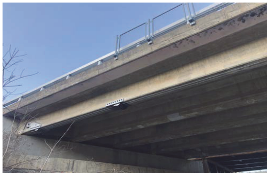
Photo 1 PSC beam girder bridge for verification
