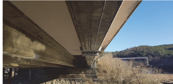
Fig. 2 External wire for strengthening the bridge
