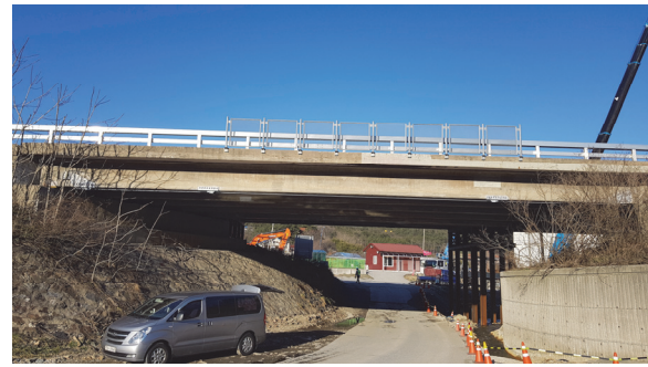
Fig. 1 View of test bridge A
