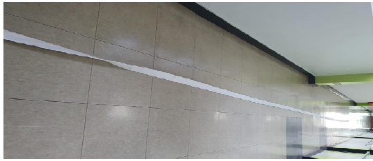
[Figure 5] Kinked state of accordion-type
