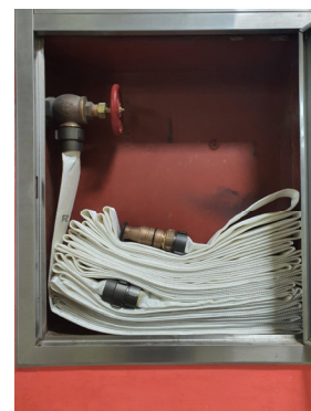
[Figure 2] Accordion-type
