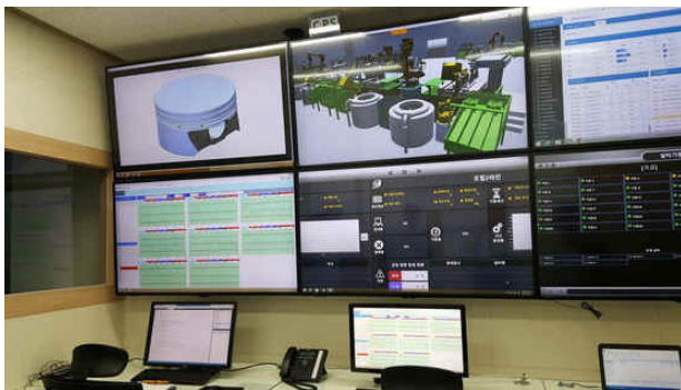
[Figure 4] Observation of smart factory at control room.
