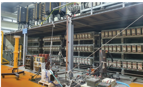
Fig. 4. Simple synthetic test facility.
