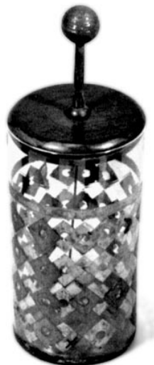
Figure 3. Sparking Leyden Jar, catalogue # 74.013.059-51 [The Bakken Museum Artifact Collection, http://oldsite.thebakken.org/artifacts/sparking-Leyden.htm ]
