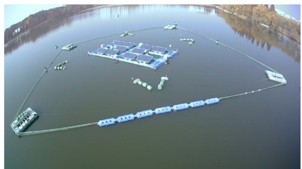
Fig. 3. Top view of the pivotless tracking type floating photovoltaic system
