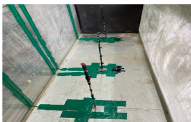
(2) PWP and accelerometer installation
