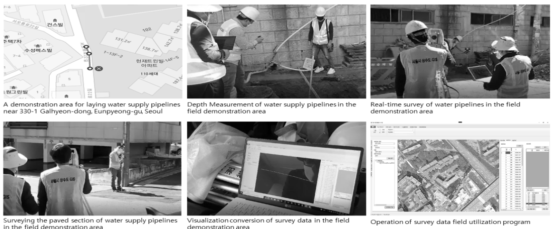
FIGURE 10. On-site demonstration of water supply pipeline laying construction from kakaomap capture, on-site still photos, and developed program capture
