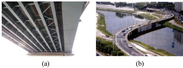
Fig. 4 Examples of representative bridges: (a) Gwangjin bridge (b) Hagye bridge
