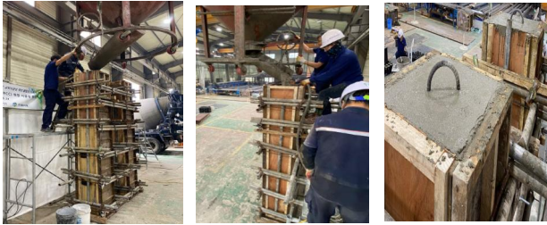
(a) Ready-mixed concrete filling
