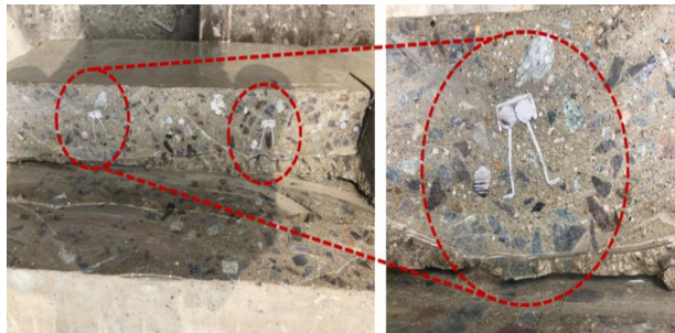
(b) Clip status check after column section cutting
