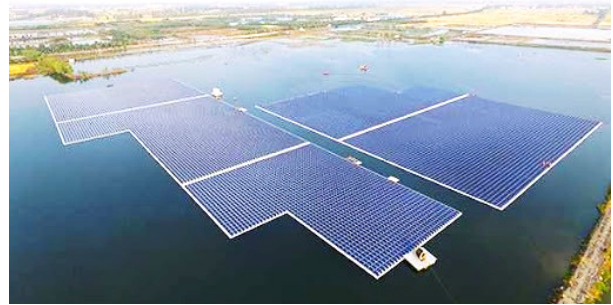
Fig. 6. Floating solar power plants 55)
