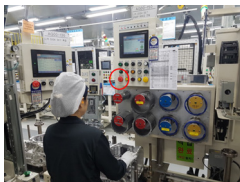
(e) Emergency Stop Device Installation.
