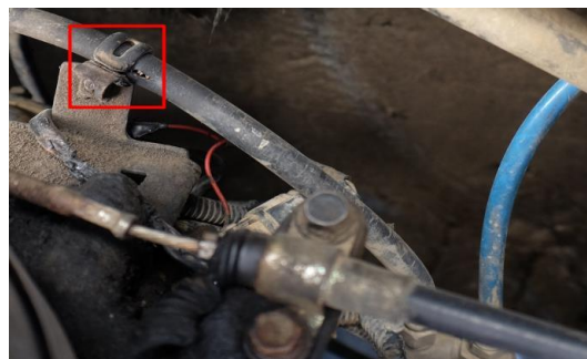
Fig. 14 A burst of the flexible hose
