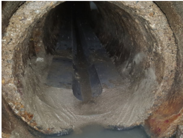
Fig. 6. Test-bed installation of complex cross section using stainless steel.
