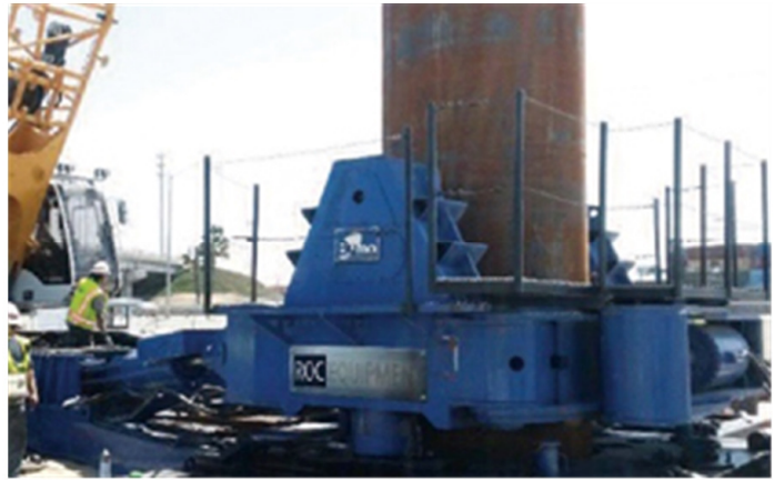
(b) Inserting step of casing
