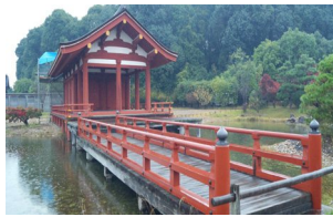
Figure 13. A Restored Building and Bridge of East Palace Garden in Heijokyo Palace
