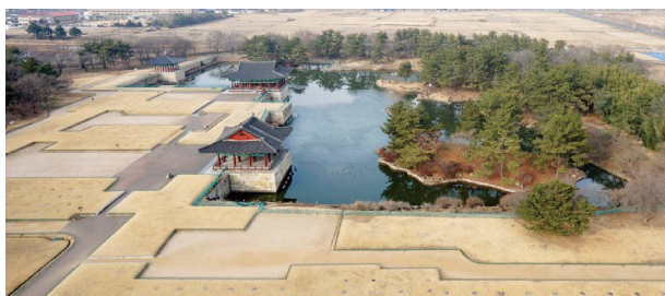
Figure 9. A Current Status of Post Restoration The Donggung Palace and Wolji Pond
