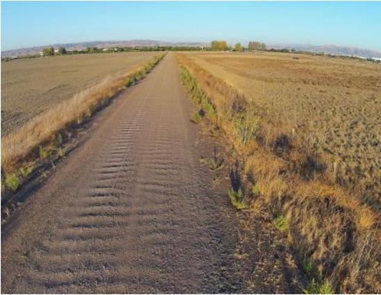
Fig. 1 Typical example of washboard road<sup>[1]</sup>
