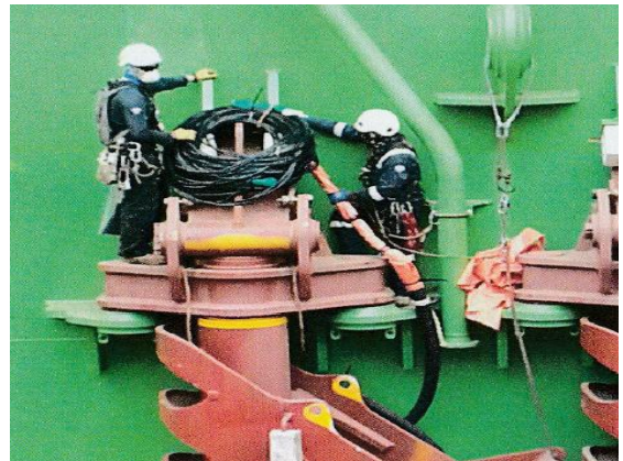
Fig. 6 Photograph of installed cable pipe
