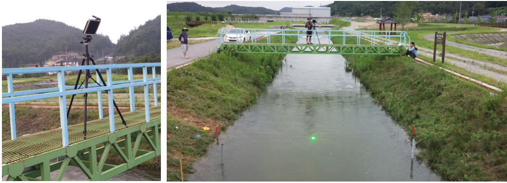
Fig. 5. MWSCM measurement on a mobile bridge located in the KICT REC straight channel
