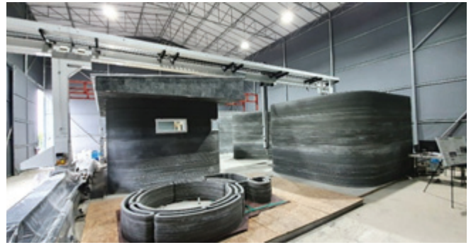
Fig. 2 3D Printing house in test-bed (KICT)
