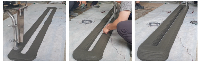
Fig. 5 Printing specimen preparation process
