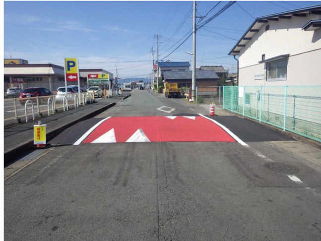
Figure 1. Example of a hump implemented in Saga-city [3]
