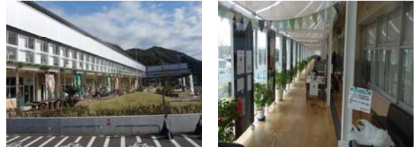
Figure 2. Hota Elementary School Remodeling
