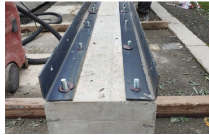
(a) Installation of lower plate
