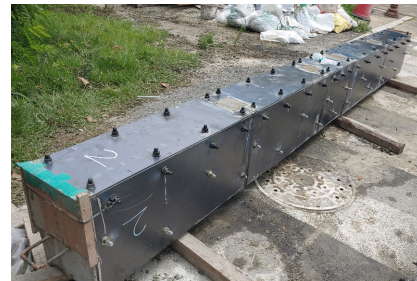
(c) Grouting of mortar
