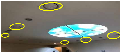
(b) The location of the ceiling thermostat
