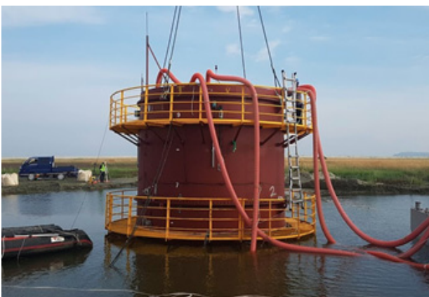
(a) The steel pipe cofferdam installation using suction
