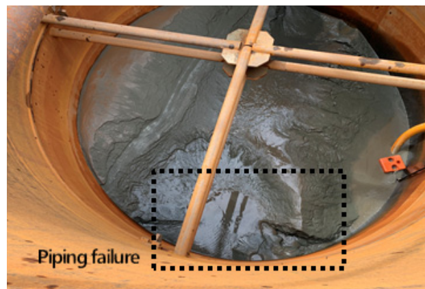
(b) Inside the steel pipe cofferdam
