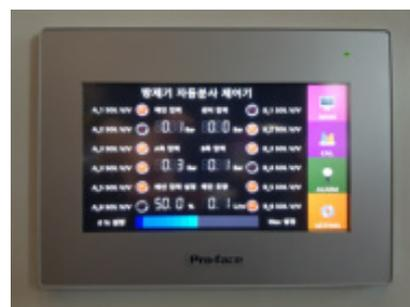
Fig. 3 Control system for valve control and operation status monitoring
