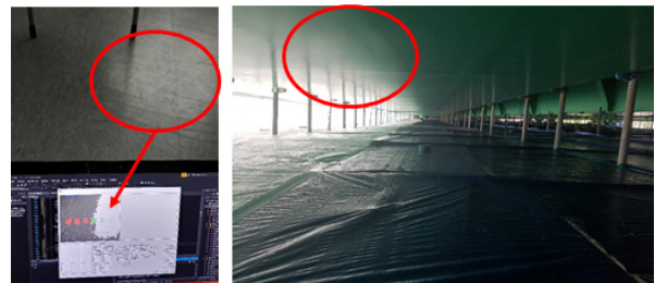
Fig. 7 Steel bridge and working environment
