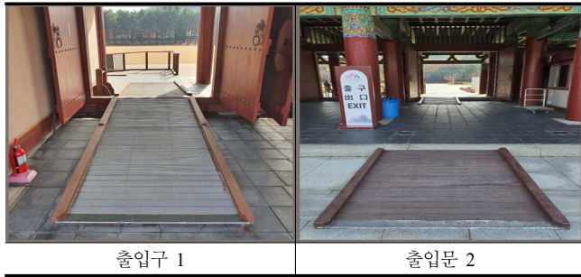
Fig. 3. Baekje Rehabilitation Complex Disabled Facilities
