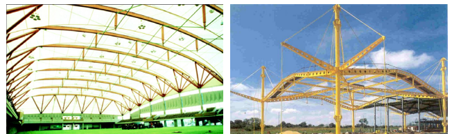
(a) Example of Tree Type Strut (b) Example of Back Stayed Cable
