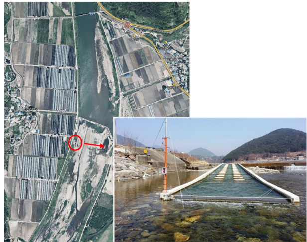
Fig. 5. Photograph of Baekgok weir and ice-harbour type fishway in Deokcheon River (after Rural Research Institute, 2015)
