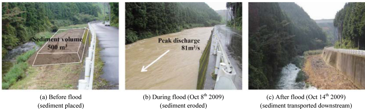
Fig. 2. Sand-gravel replenishment by high-flow stockpile method in the Nunome River, Japan (Ock et al. , 2013b)
