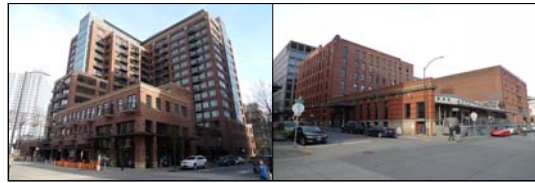
Fig. 15. Mixed-Used Renovated Building
