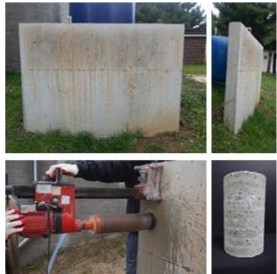
Figure 3. Core sampling of mock-up wall
