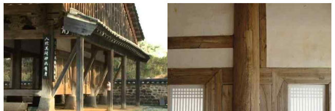
Figure9. Application of Myochim theory for Nonsan Donamseowon, eongdodang (Left:Supplemented eave, Right:Vestige of a column)
