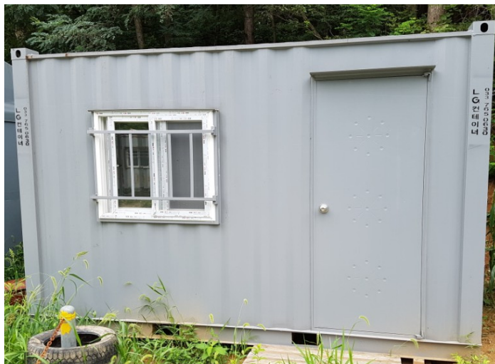
Pilot container for anaerobic digestion
