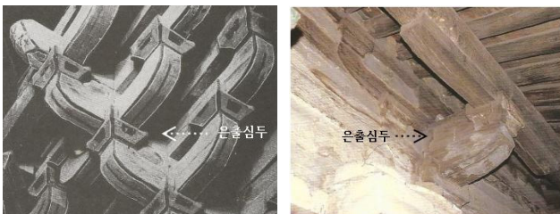
Fig. 8. Eunchulsimdu(隱出心料) system example
