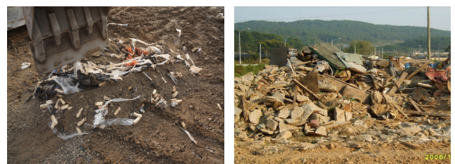
Fig. 9. Panorama of mixed construction waste
