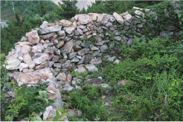
Fig. 3 Heuksando fire signal site (source : Dadohaehaesang national park west office, 2013)
