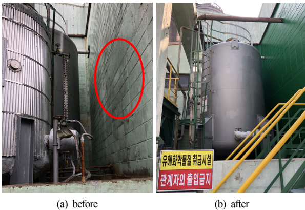
Fig. 8. Acid resistant painting treatment.
