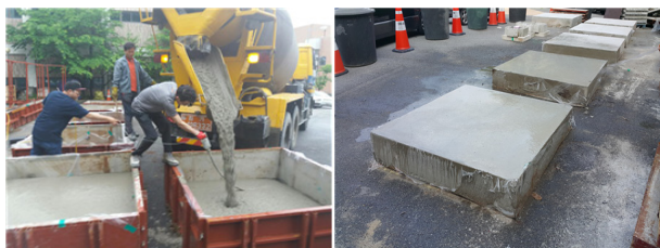
Figure 2. Preparation of specimens
