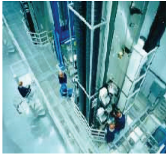
Fig. 5. The structure of the draw tower
