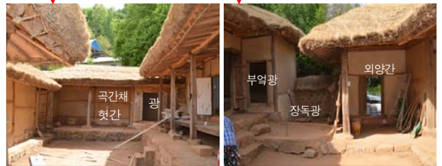
Fig. 13. Attached buildings of the house
