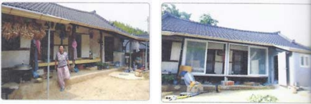
Fig. 9. Work of window and door in front of house
