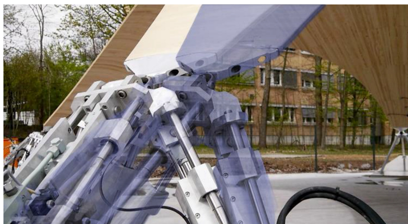
Figure 2. Stuttgart SmartShell movement of bearings; Source: ILEK, Gabriele Metzger.
