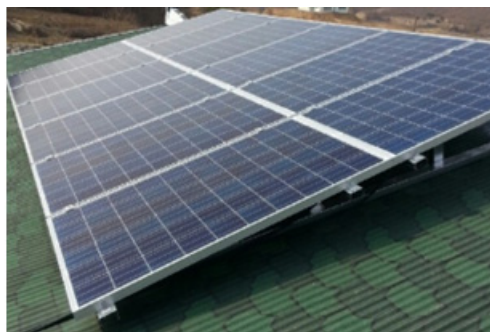
Fig. 1 Semi-integrated with air duct behind
