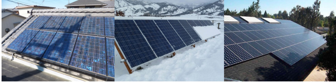
Fig. 1 An example of the mismatched situation caused by partial shadow in PV array
